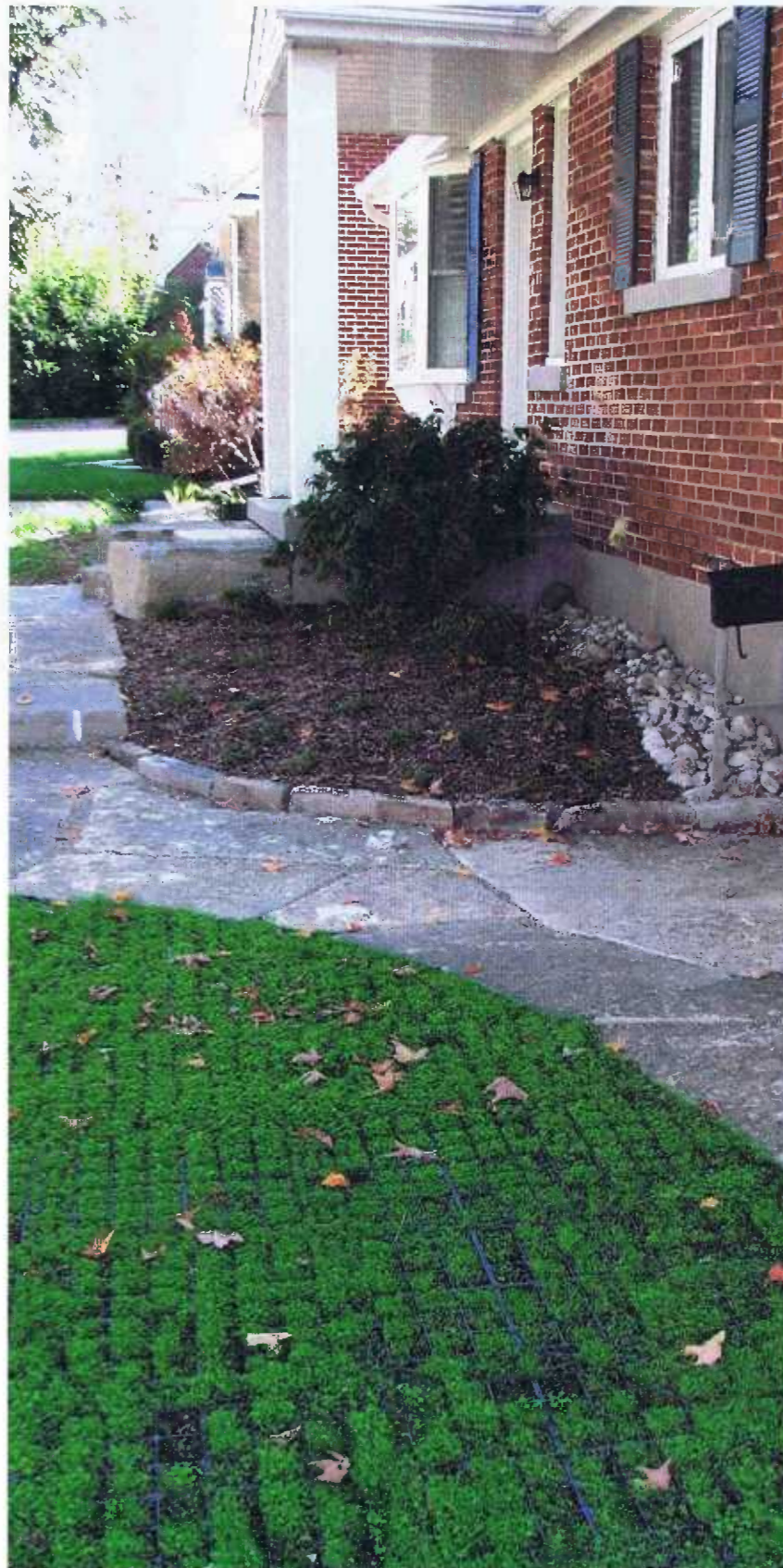
Showing through the European micro-clover used as a groundcover at this Waterloo home are the plastic grids that provide support for parked vehicles.
